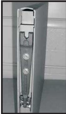
Figure 1a: Centering Bracket in top of door.
