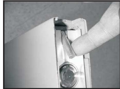
Figure 1b: 218 Pivot in bottom of door.
