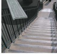
TYPE 103 - Nose 3/4" x 3/4". (19.05 mm x 19.05 mm). Chief use: as structural treads with bent-plate risers or as nosings full width of stair.
