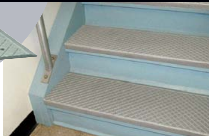
TYPE 116A – GREAT FOR EXISTING INDUSTRIAL STAIRWAYS AND/OR LANDINGS.
